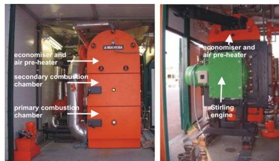
Figure 8: Pictures of the small-scale CHP pilot plant with a 35 kW<sub>el</sub> Stirling engine
