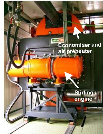
**Figure 7:** Picture of the small-scale CHP plant based on a 75 kW<sub>el</sub> Stirling engine – backward view
