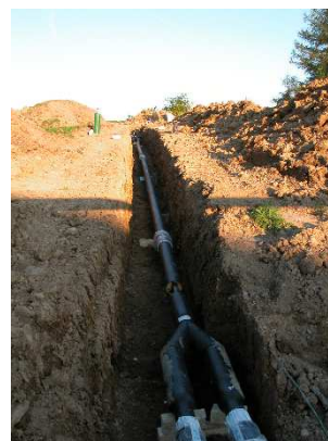
Laying of district heating pipes
