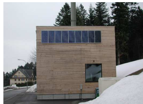
Exterior view of a biomass heating plant
