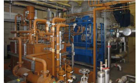
Kufstein / A 6.5 MW el steam turbine
