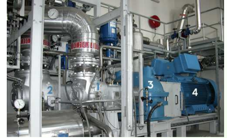
Hartberg / A 0.8 MW el steam screw-type engine
