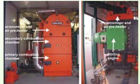
Reichraming / A 35 kW el Stirling engine
