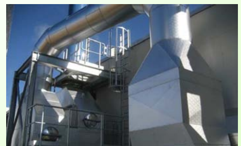
Wörgl / A Flue gas condensation
