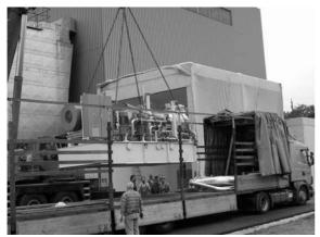
Figure 5: Unloading of the screw-type engine module
