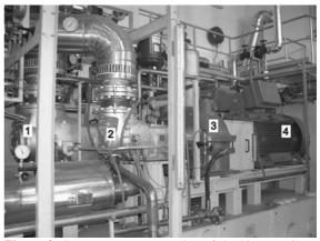
**Figure 8:** Screw-type steam engine of the biomass CHP plant in Hartberg (net nominal electric capacity: 710 kW<sub>el</sub>)
