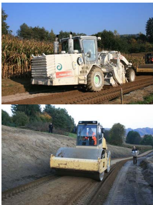
Figure 8: Mixing of the binder with a rotary hoe and subsequent compacting with a roller compactor
