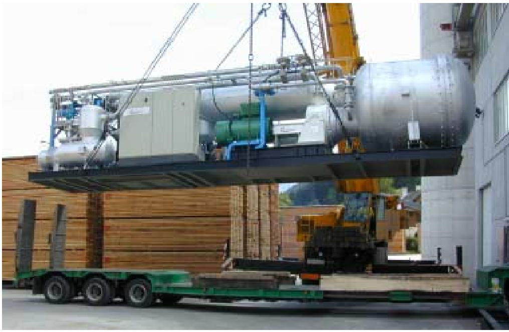
Figure 4: Delivery of the ORC plant
