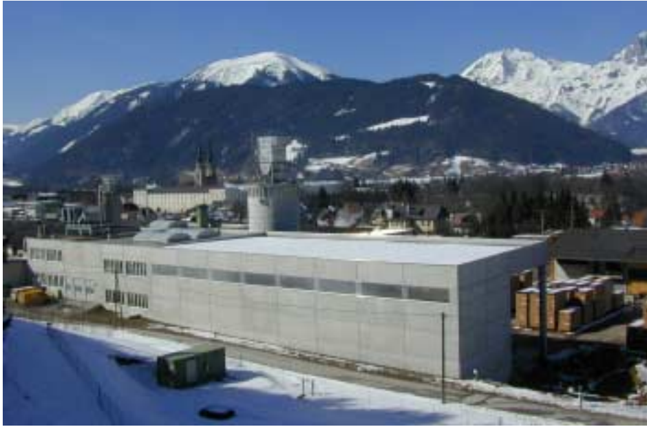
Figure 1: View of the Admont CHP plant with fuel storage hall and boiler house
