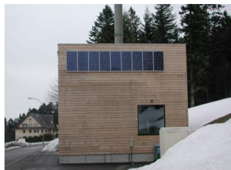
Exterior view of a biomass heating plant
