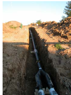
Laying of district heating pipes
