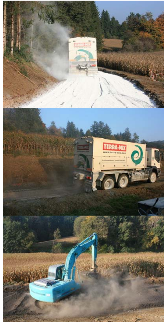
Figure 7: Application of the individual binders used in the field test
