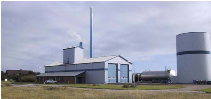
Figure 14. Picture of the updraft gasifier plant in Harboere (DK)
