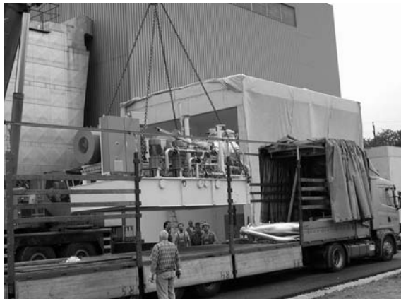
Figure 5: Unloading of the screw-type engine module
