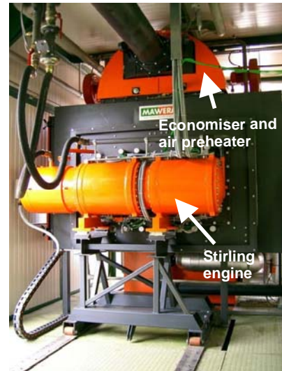
Figure 7: Picture of the small-scale CHP plant based on a 75 kW el Stirling engine – backward view
