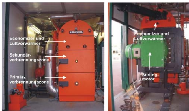
35 kW el pilot plant based on a Stirling engine
